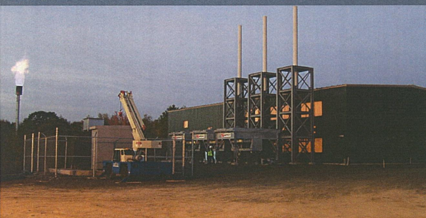
Landfill Gas Power Plants
